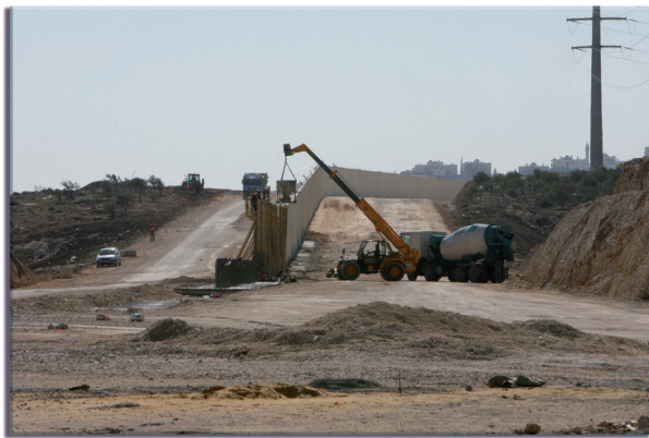
Road No. 70 (under construction) will run parallel to the wall. Jan 2007.
