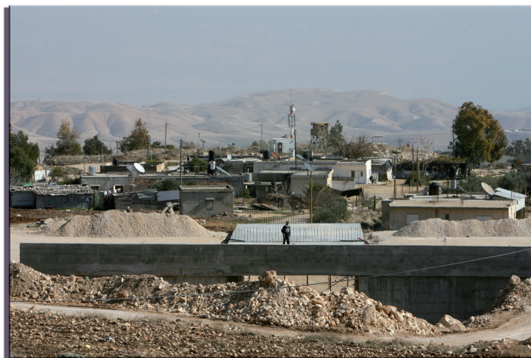
The wall in the Al Fheidat neighborhood will separate it from its center in Anata. The only ingress or egress for Bedouin community is via the underpass below settlement Road No. 70. Jan 2007.
