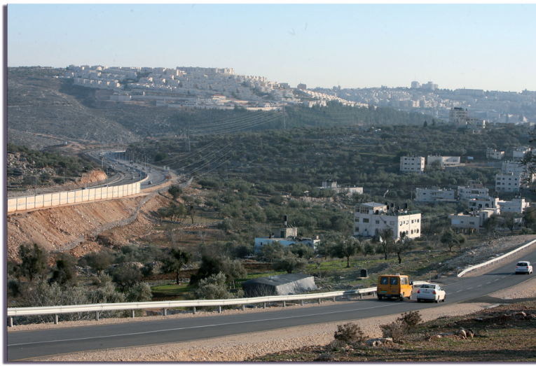
This alternative road constructed west of Road No. 404/4 will connect Beit Hanina Al Balad to Ramallah and end its link with Jerusalem. Jan 2007.
