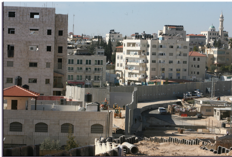
The wall under construction in Dahiyat Al Bareed. Jan 2007.
