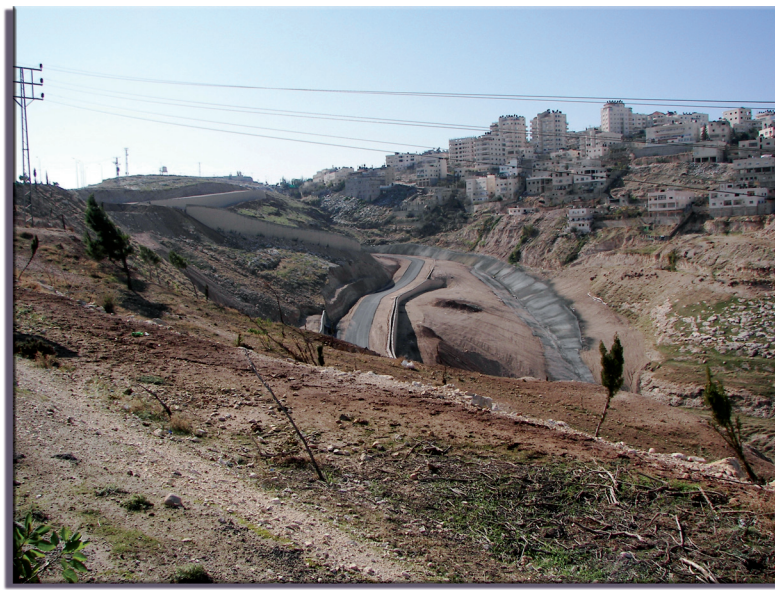
A road tunnel under construction northeast of Al Eizariya will connect Al Eizariya/ Abu Dis enclave with the Shu'fat RC/ Anata enclave replacing the territorial contiguity between south and north West Bank with a transportation link. Jan 2007.
